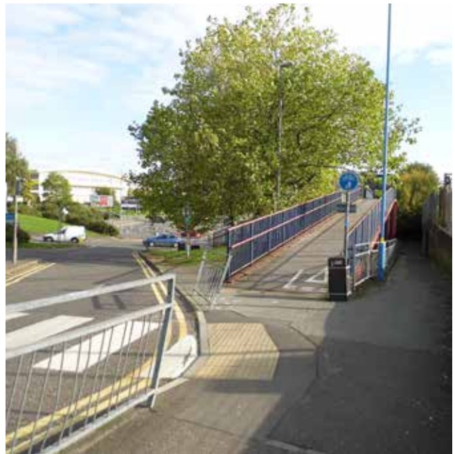
It is not clear that pedestrians need to go under the bridge to find the route to the town centre
